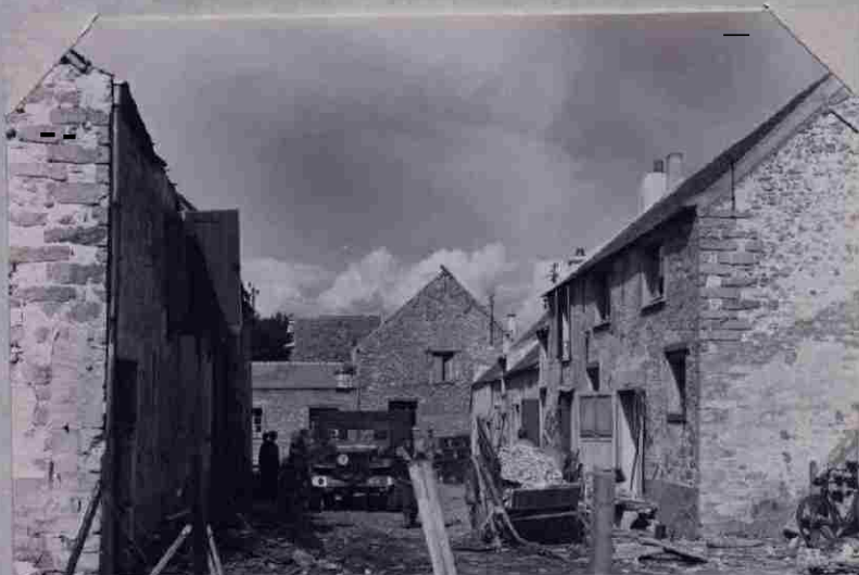
Exh #3-C-Sept 1944-View of courtyard at Headquarters during the cleaning-up operations.
