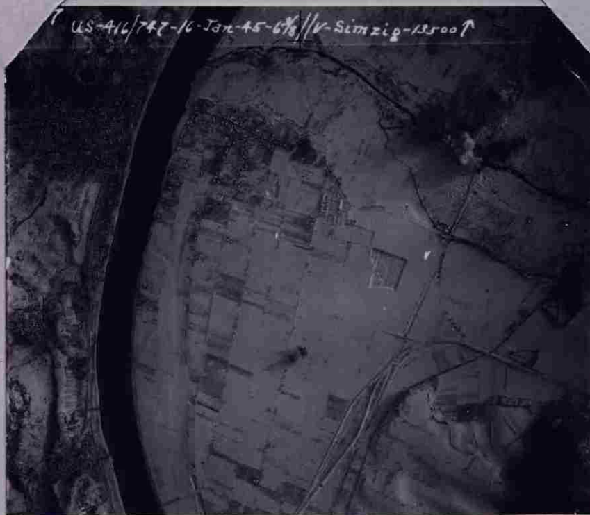
Exh #17-Jan 45-The Sinzig railroad bridge remains standing, but the bombs severed the tracks approaching on 16 January.
